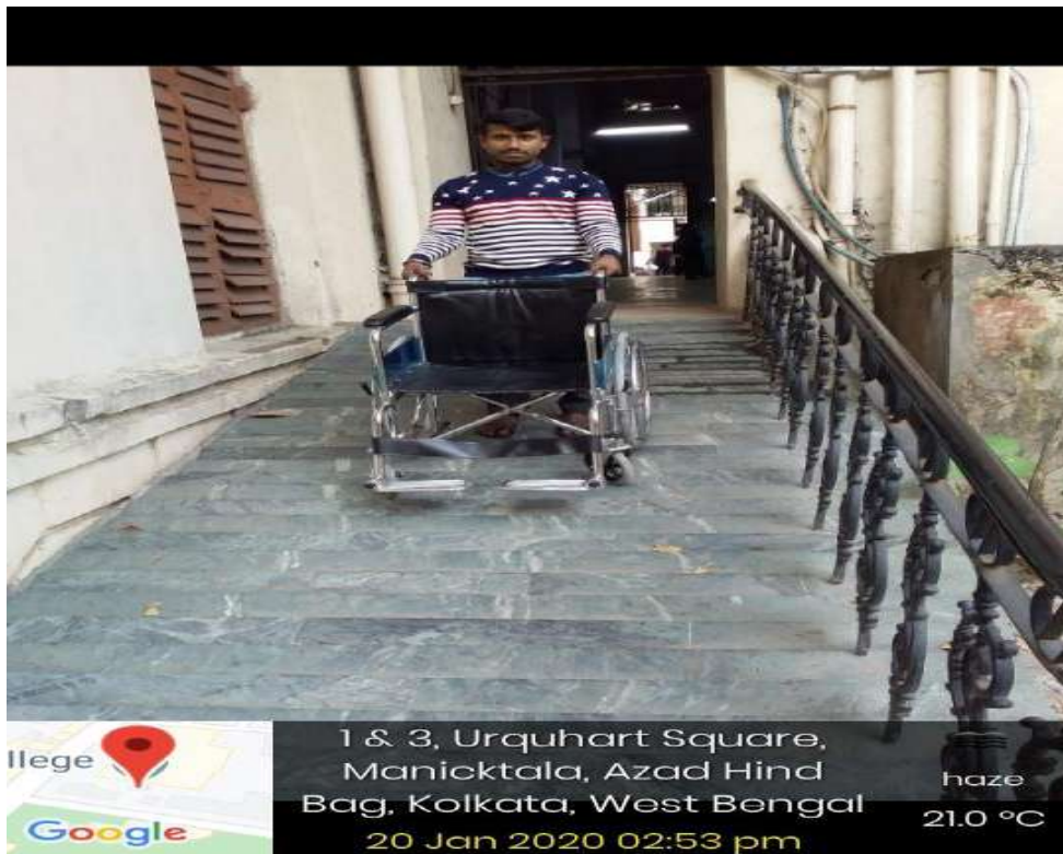
RAMP AND WHEELCHAIR
